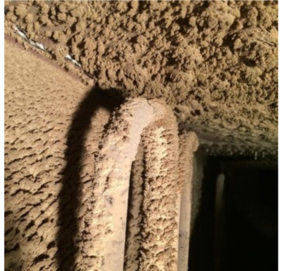
Ash deposits in the L1500 furnace.
